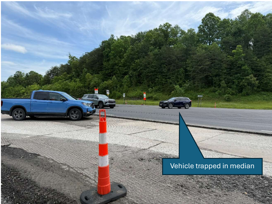
Ames Heights Road/Lansing-Edmond Road Intersection – Looking Northeast
