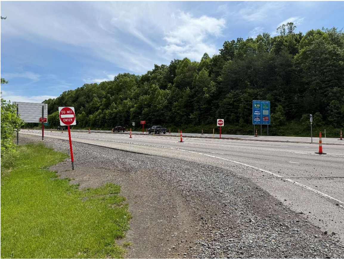
Fayette Mine Road/Burnwood Campground Drive Intersection – Looking north along US-19
